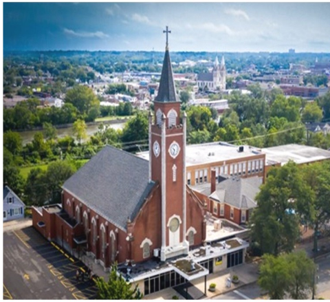
706 North Broadway Street Joliet, Illinois 60435
