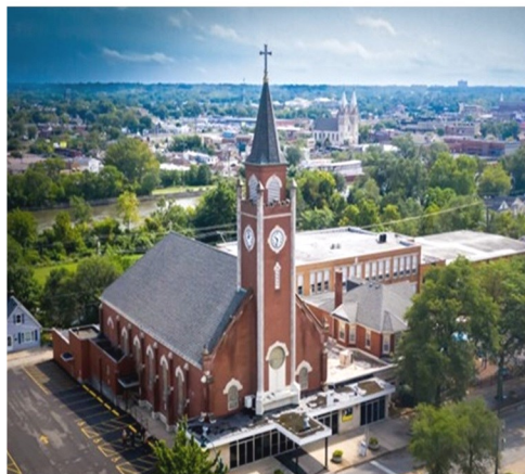
706 North Broadway Street Joliet, Illinois 60435
