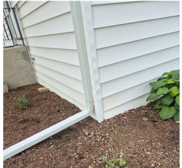
HC Rectory Downspout Repair
