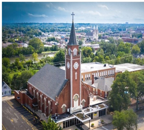
706 North Broadway Street Joliet, Illinois 60435
