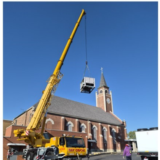
Removal of old chiller at SMN
