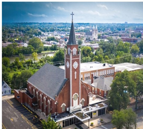
706 North Broadway Street Joliet, Illinois 60435
